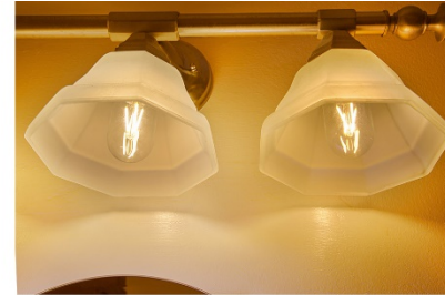
T14 LED bulbs in bathroom vanity light fixture
