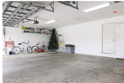
T8 LED bulbs in garage tube light fixture
